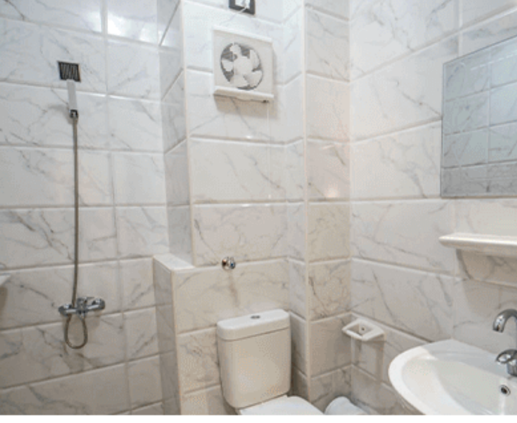
Adding bathroom fans
